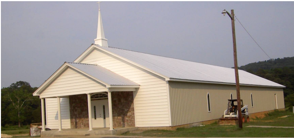
Friendship Baptist Church construction (July, 2008 photo)
