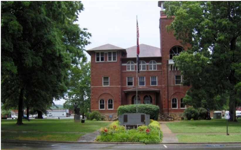
Rhea County Courthouse
